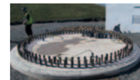
Concrete foundation ready to install the turbine
