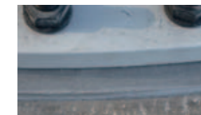
Hardened Masterflow® 9300 ExagROUT & pre-stressed bolts
