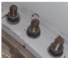
Hardened MASTERFLOW 9300 ® ExagROUT & pre-stressed bolts
