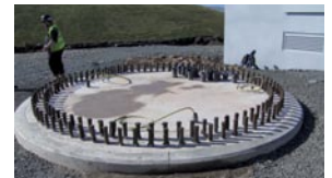
Concrete foundation ready to install turbine
