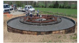
Concrete being poured into on shore foundation
